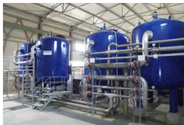
Water treatment in sand and coal filters
